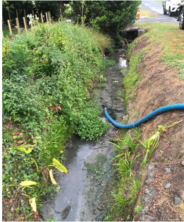
Figure 10. Domestic wastewater discharge to waterway being removed via sucker truck
