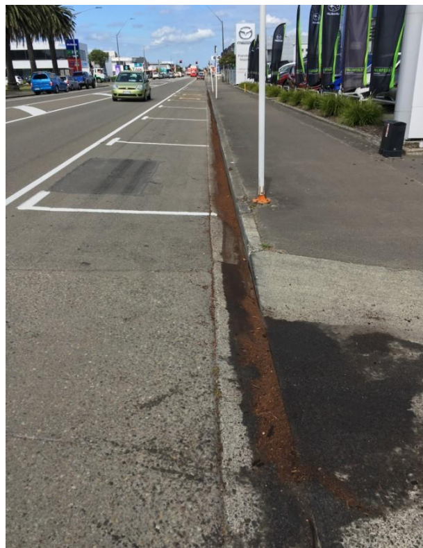
Figure 7. Oil spill to stormwater network
