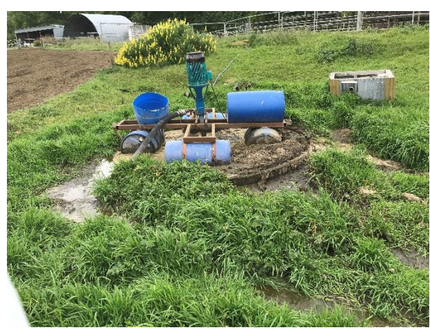
Figure 6: Sump Overflow
