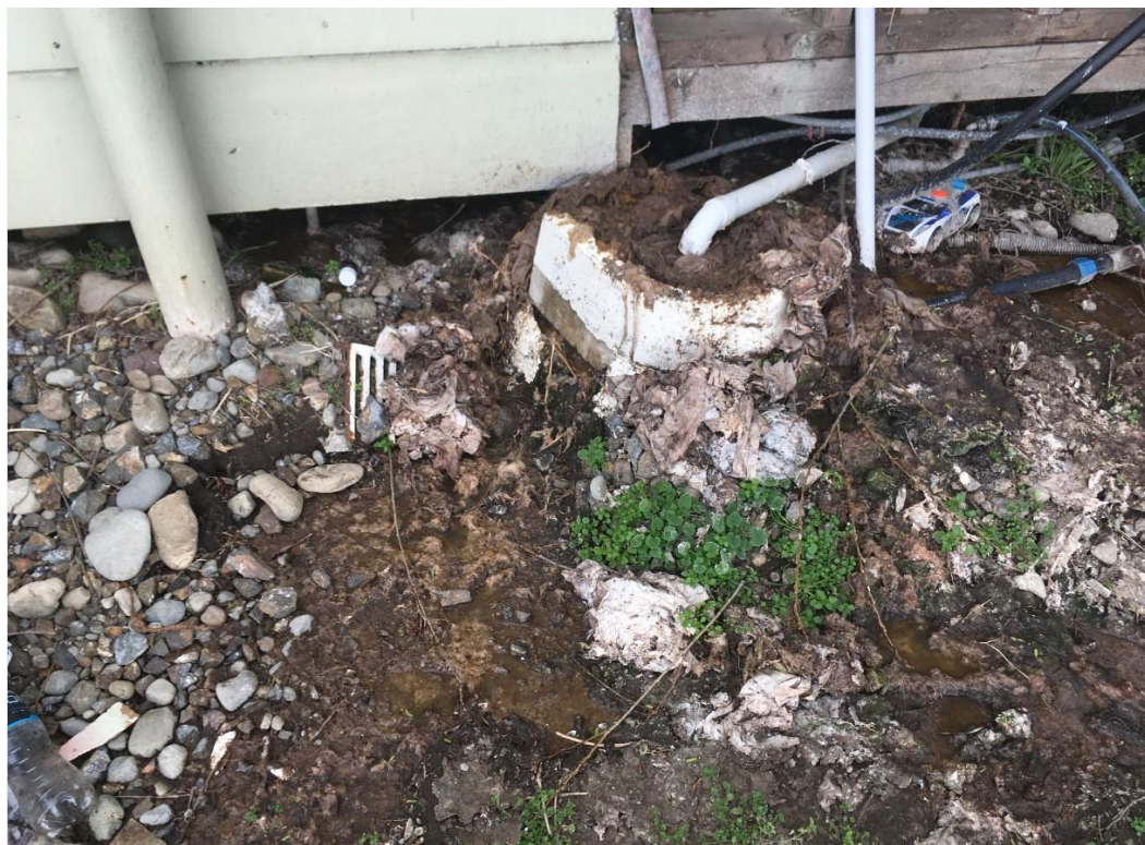
Figure 9. Domestic waste system discharge
